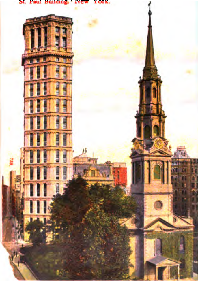
St. Paul Building, New York.
